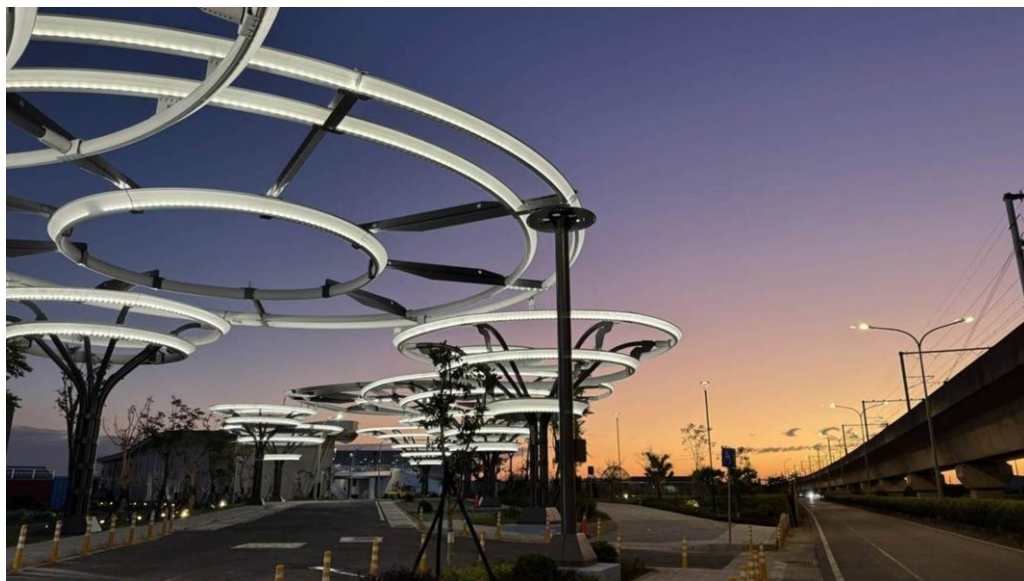
Bao-Ding Reclaimed Water- Taoyuan North District Water Reclamation Center 寶鼎再生水-桃園北區再生水中心
